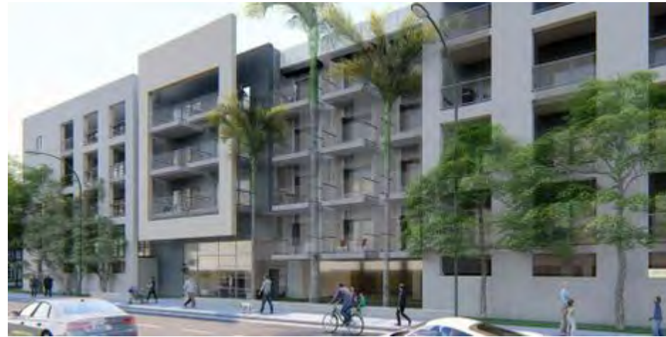
4 7322-7340 Topanga Canyon Blvd 7334 Topanga Canyon Blvd Canoga Park, CA 91303
